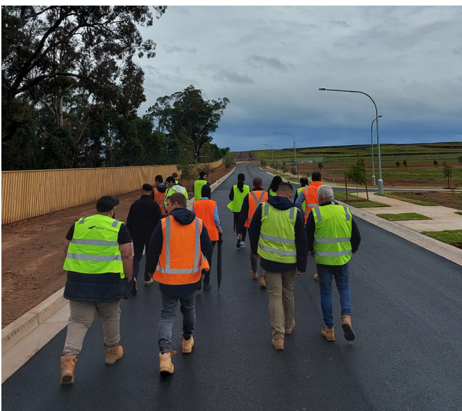
Project team doing a site walkthrough and inspection
